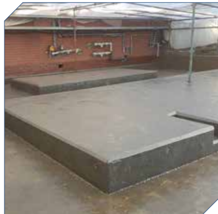
Following application of Corrofill E.
