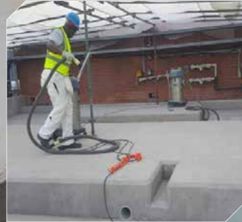
After application of 1st coat of Plasmet ECP Primer.
