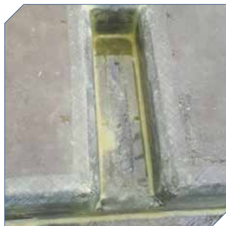
Application of Plasmet AR3 in progress.
