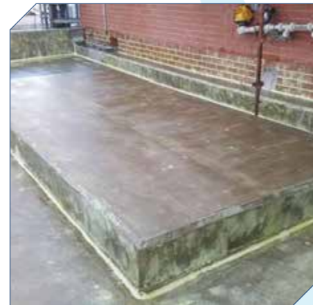
Application of 2nd coat with C-Glass fibre laminate.
