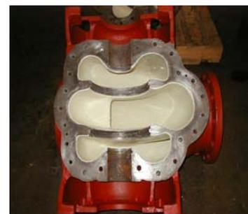
*Corrocoat branches worldwide have been successfully refurbishing pumps for almost three decades, returning damaged and corroded equipment to 'as new' condition.*
