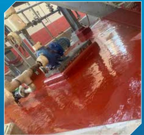
Shortly after reviewing Corrocoat USA's corrosion assessment report, the client hired Corrocoat USA to supply and apply our Plasmert AR3 lining system, to refurbish the surface and protect against continual immersion. Some work was completed using pre-coated fiberglass sheets while the building was running, and then applied directly at a later stage to the prepared concrete, while the client addressed the root causes of their corrosion problems.
