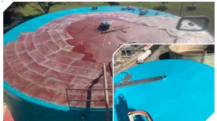
The surface was then primed with Plasmert ZF (red) ahead of using Epoxy Laminating Resin and quadriaxial fiberglass mat to laminate a composite fiberglass layer across the entire tank roof. The team then chose a suitable polyurethane topcoat to offer UV protection in a colour that matched the remainder of the tank. The client was extremely impressed with the final result and the quality assurance and will continue to work with Corrocoat US on future projects.
