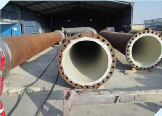
As part of a series of initial projects, a number of pipespools required repair and restoration from corrosion damage at a seawater injection plant. The project ran over 9 months and Polyglass VEF was the primary coating system used throughout. Polyglass VEF was the ideal coating system for this project, protecting the spools from future corrosion damage from seawater and in turn extending their service life considerably.
